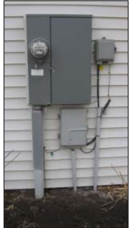
Figure 1-15-a. 200 Amp surface mounted meter socket.
