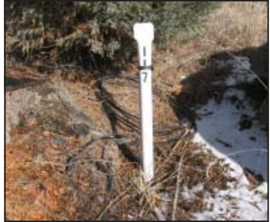
Figure 1-3. Service stub out.
