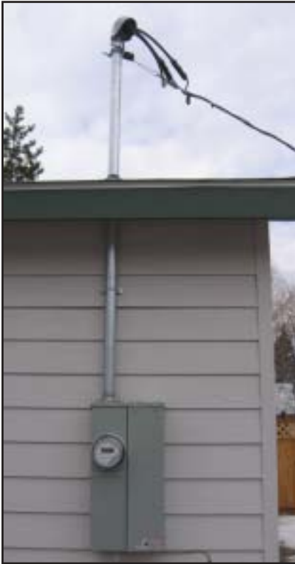
Figure 1-11a. Surface mounted meter socket example.
