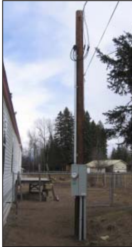
Figure 1-12a. 100/200 Amp overhead service.
